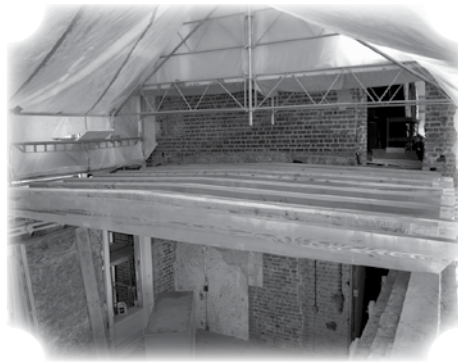
RESTORED BEAMS, WRAPPED TO SUPPORT THE SERRATED ROOF OF ONE OF THE WINGS
