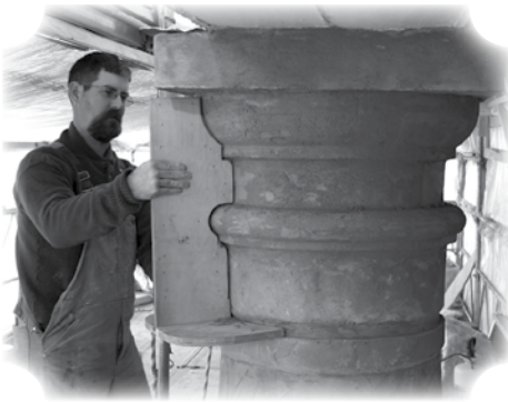
A CONTRACTOR CAREFULLY CHECKING A TEMPLATE OF THE HOME'S COLUMNS.
